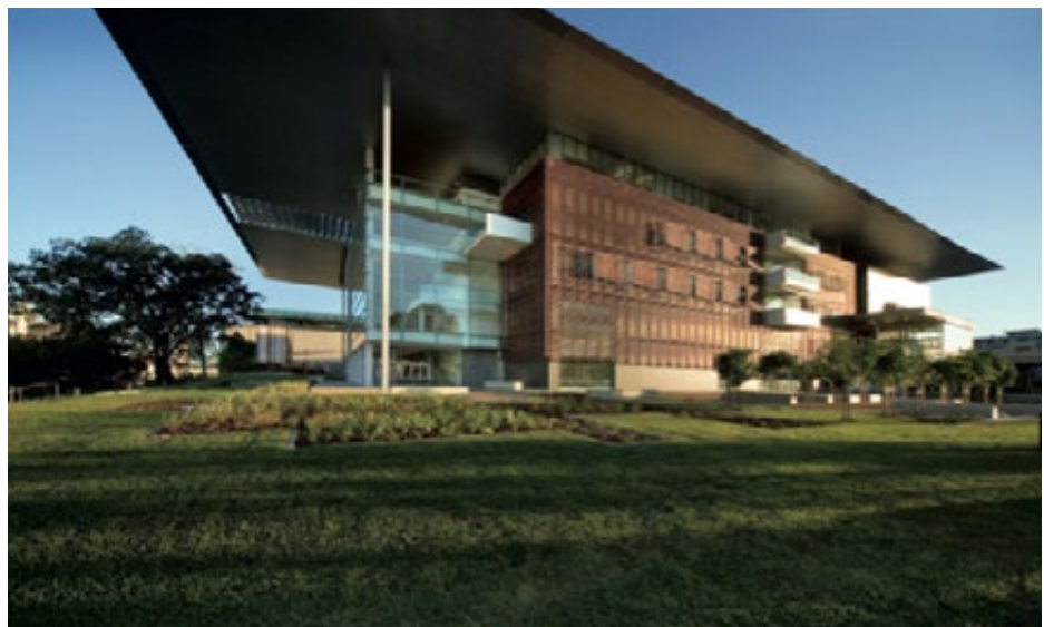
View of gallery from north west. Large timber screen to administration and curatorial areas. Photograph by John Gollings.
